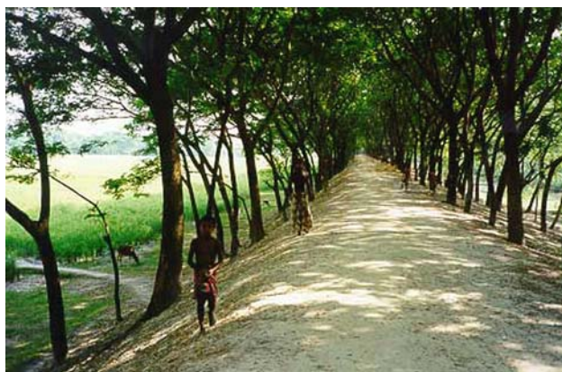
Fig. 7 A typical cyclone-proofed access route in the south–west coastal region of Bangladesh (Photo: M. Karim)
