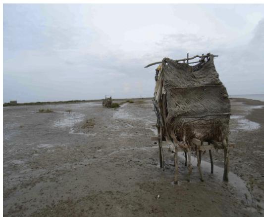
Picture 2. Community toilet in Keti Bandar.
