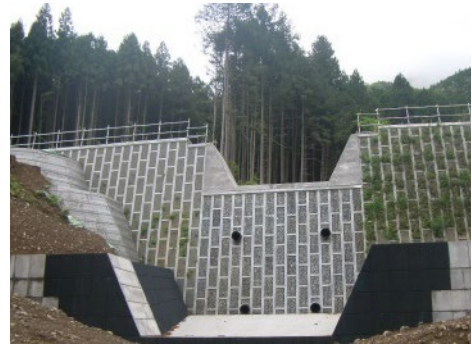
Erosion control facility
