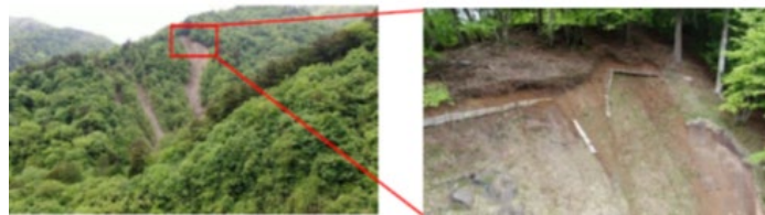
A distant view of a collapsed area (Photo taken by a drone)
