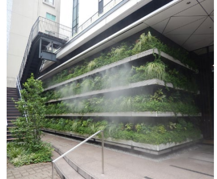
Example of installation of fine misting devices (OASE Shibaura, Minato-ku)
