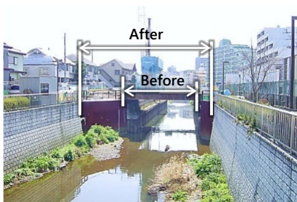
Revetment construction (Shakujii River)
