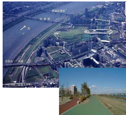
High standard embankments
