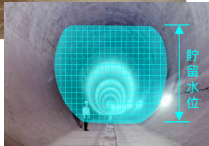
Underground discharging Channel
