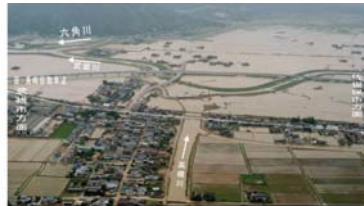
Inundation of Route 34 during a flood in July 1990
