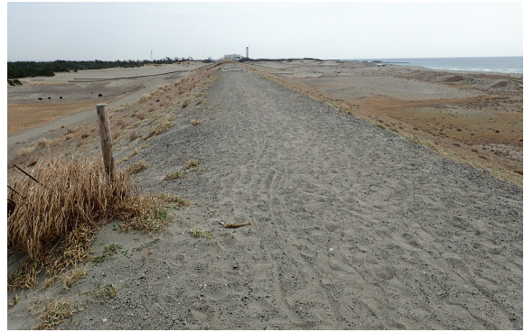
Figure 12. A coastal dike in Hamamatsu city, Shizuoka, located at D in Figure 5. Top and both sides of CSG dike were covered by soil.
