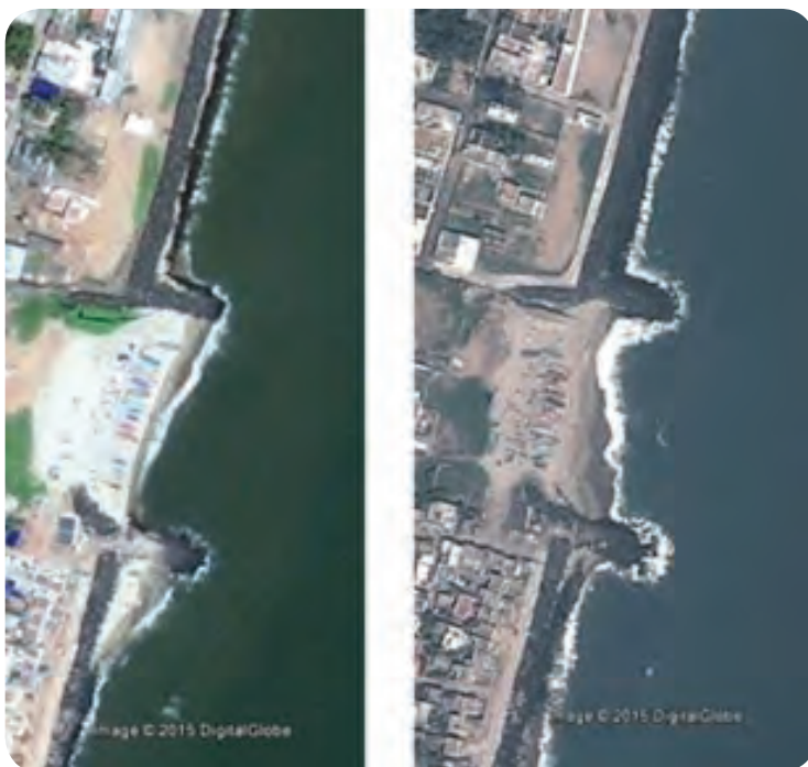
Figure 22. Seawall with Gaps and Short Groynes on either side of the Gaps, Puducherry
