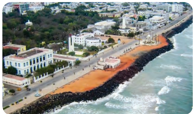
Figure 7. Pondicherry Beach before erosion (top left) and the current rock seawall and ineffective groynes along the shoreline with the degraded seawall
