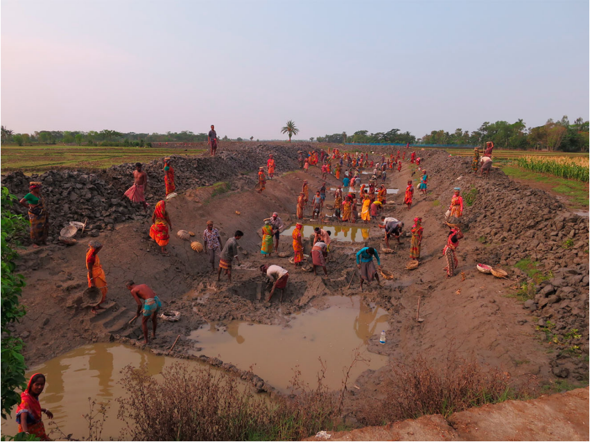
Figure 2. Canal excavation in 'Nodi', May 2015 (Source: Author).
