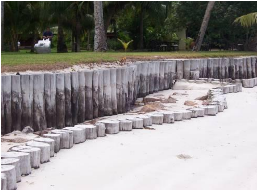
Figure 74: Existing Protection Measure on Praslin (Soft Technology)
