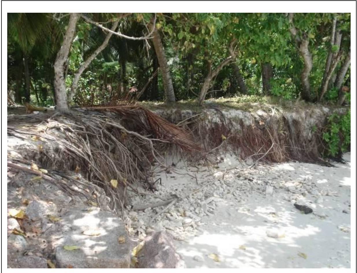
Figure 69: Coastal Erosion at the Anse Kerlan Beach (April 2007).
