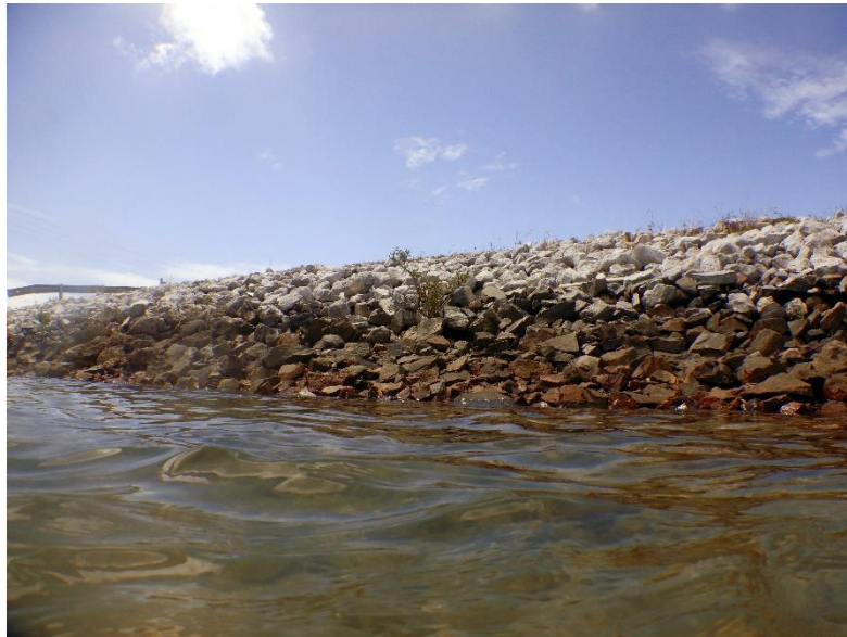
Photograph 2. Riprap shoreline along the Intake Location Survey Area.
